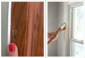
Caulk around windows where caulking is cracked or missing or between the trim and the wall if gaps exist.
